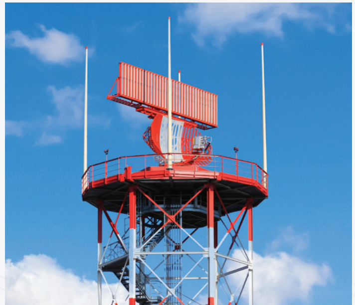
Co-mounted MSSR and passive ADS-B system
